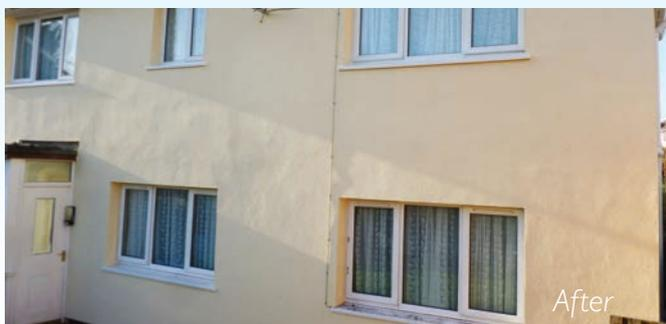
In 2014, we launched a pilot scheme involving four properties in Somerton. We installed external wall insulation, renewed roofline works, extracted the cavity wall insulation, cleaned the cavities and made various internal repair works. This pilot showed us the extent of the issue in some of our oldest stock, and so we have appointed Mi-Space to carry out a programme of work to more homes.
